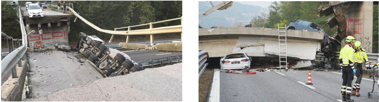
Fig. 1: Collapsed Bridge in Italy [NfS16], [MB16]
