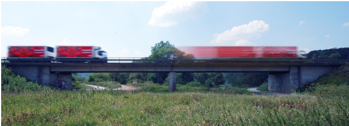
Fig. 2: Test Bridge “BW70”, Baunach
